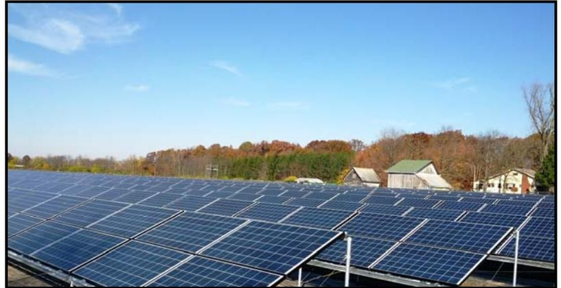
Located on the southwest edge of campus near the football and soccer stadium in Urbana, Ohio, the array consists of 2,128 solar photovoltaic modules which contribute approximately 15% of the school's energy needs. Most important to the university is that the array serves as a visible example of the school's commitment to sustainability.
